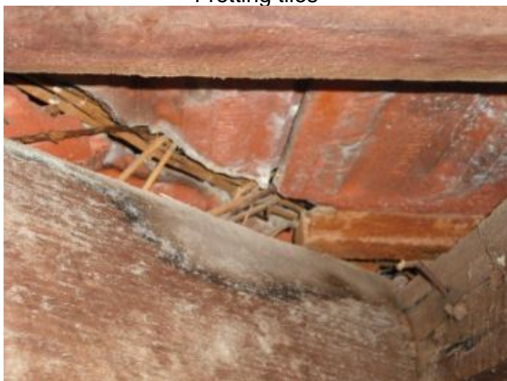
Vine in roof space
